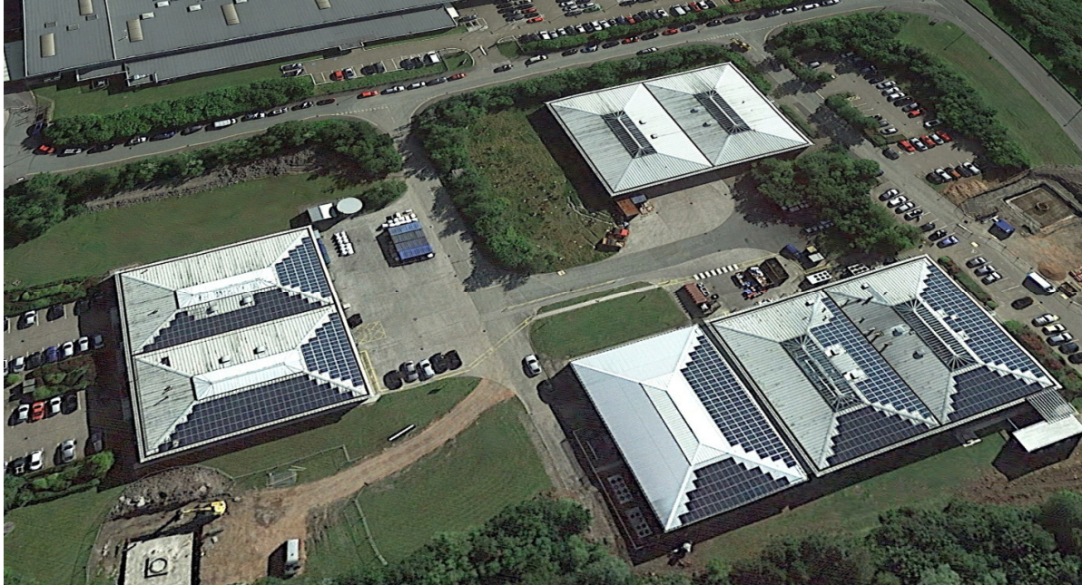
An aerial view of the Eurocaps factory, showing solar PV panels on 2 of their 3 buildings
