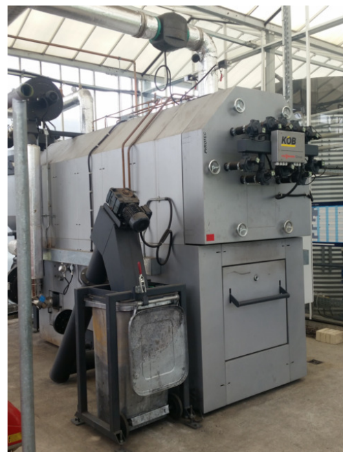
Viessmann (KOB) Pyrtec 720kW wood chip boiler
