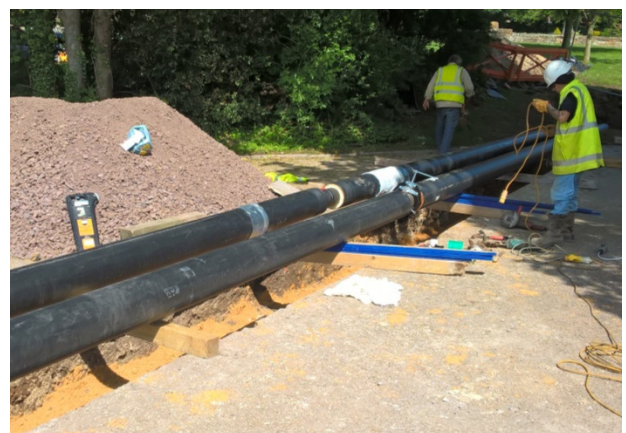
DN150 steel DH pipe installation at Clayesmore School
