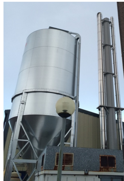
Pellet silo & flue mast at Raigmore
